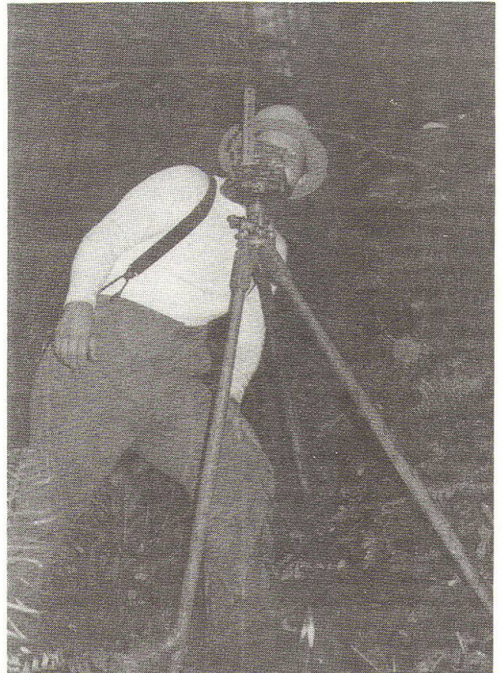
(Friday morning, August 9, United States Deputy Surveyor, Denny DeMeyer gives line with a solar compass.)
