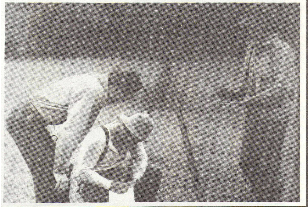
Picture lower right - Friday A.M., August 9; Tom Starr and Royce Hill trying to remember their chaining calls of the morning run. Note leather tally counter on Tom's belt, Royce holding Gunter's chain and chaining pins, and solar compass in the background.
